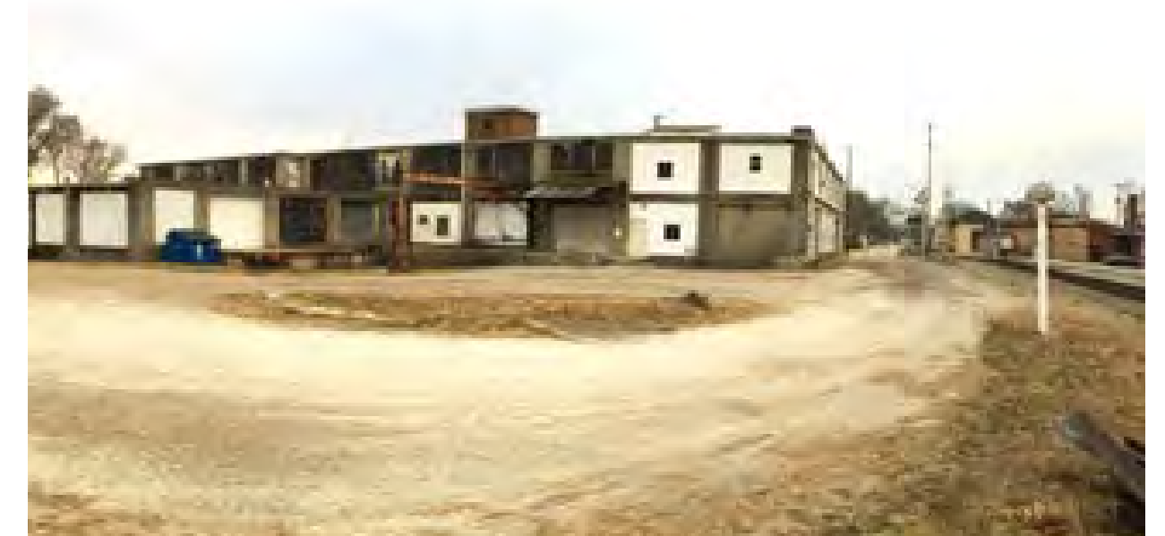
FORMER HOBART CABINET BUILDING, TROY, OH
