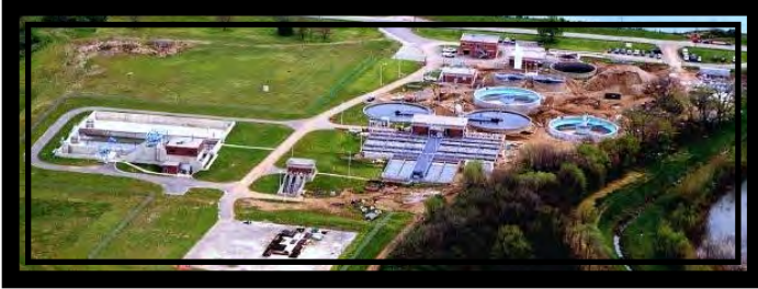
Troy Wastewater Treatment Plant 1400 Dye Mill Road
