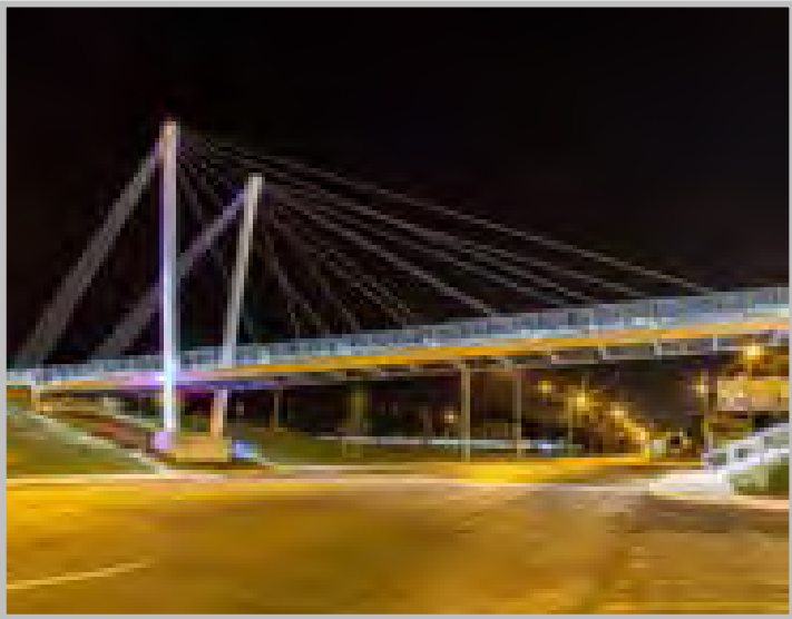
Example of Architectural Lighting on Bridge
