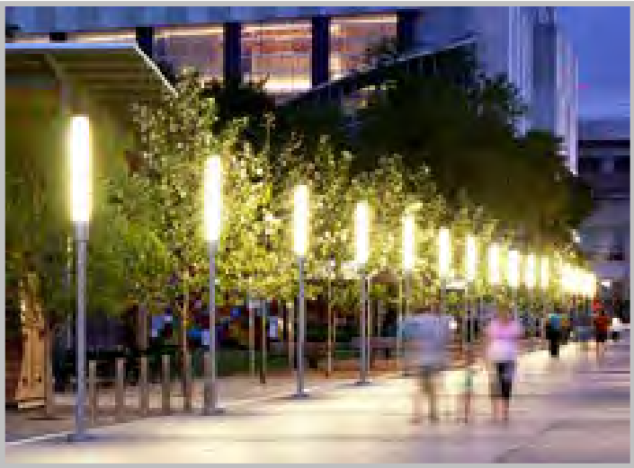
Light Fixture Example for Landings
