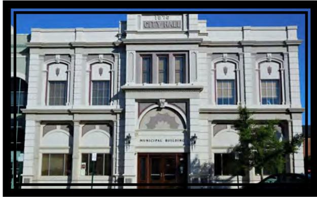
Troy Municipal Building 100 South Market Street
