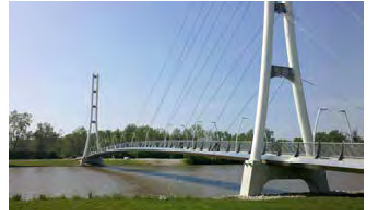
PEDESTRIAN BRIDGE EXAMPLE
