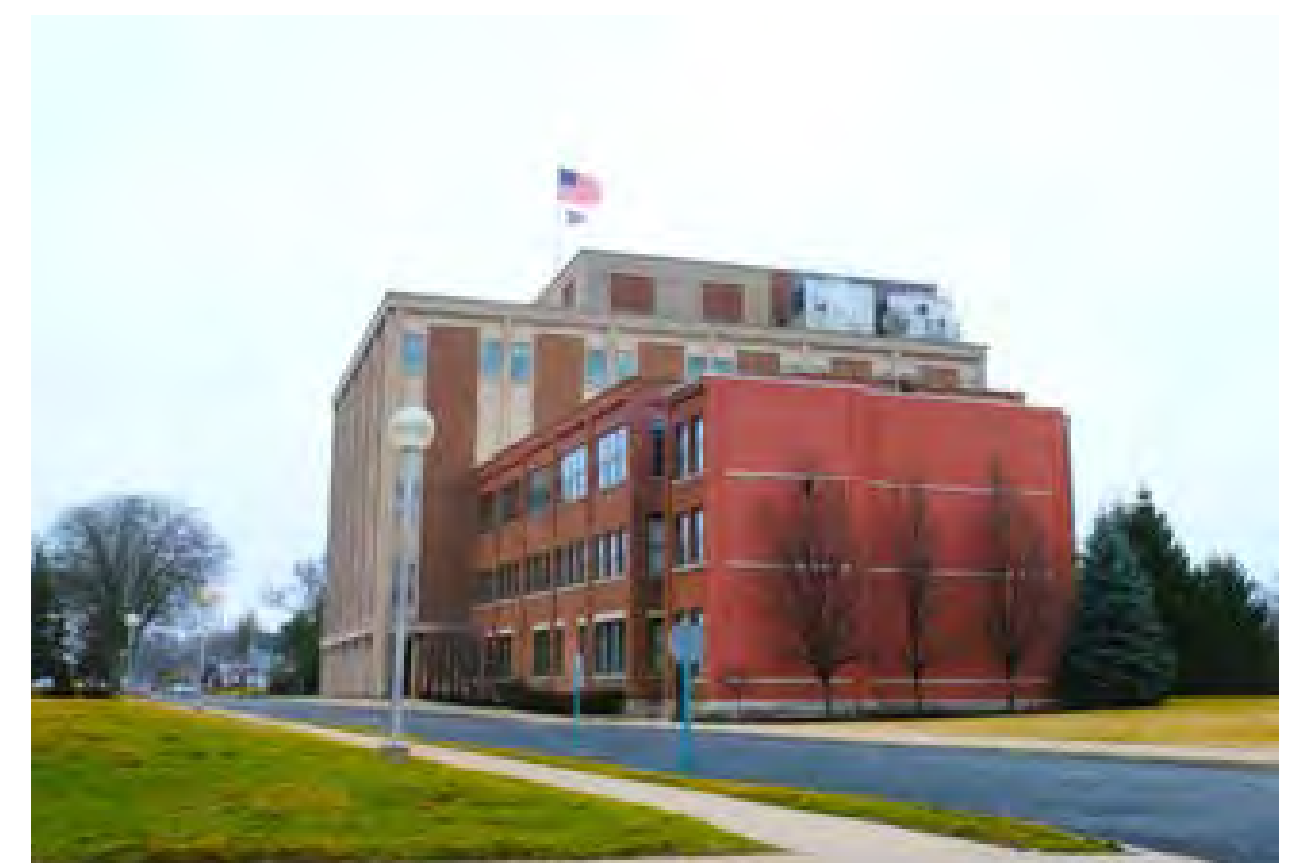
FORMER HOBART RIDGE AVENUE CAMPUS, TROY, OH
