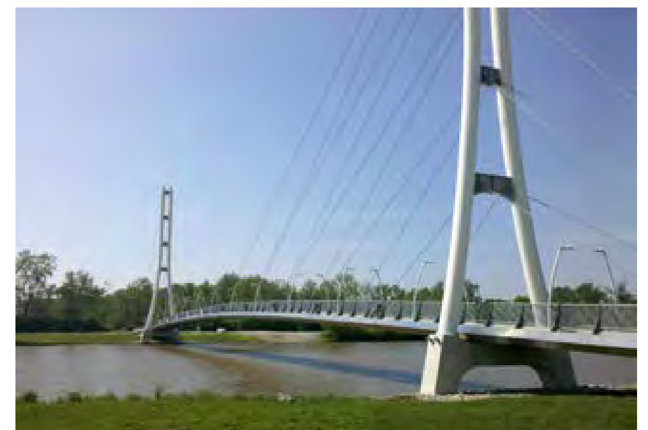
PEDESTRIAN BRIDGE EXAMPLE
